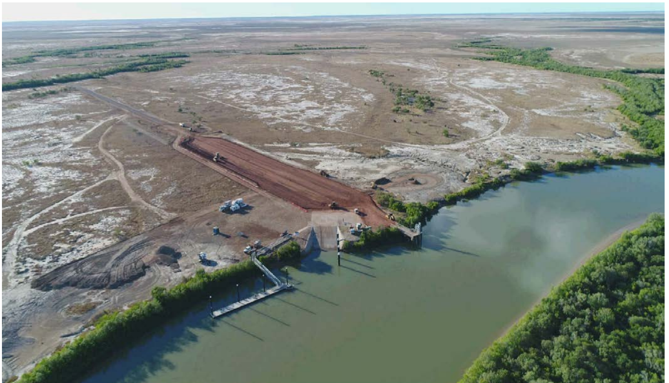
Image: construction of the Burketown Wharf Boat Ramp and Car Park.
